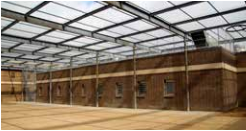
CALCASIEU PARISH PRISON ADDITIONS
