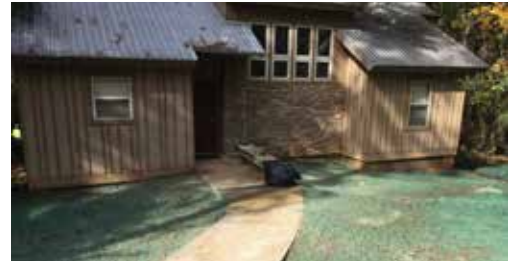
STBSP CABIN STABILIZATION PH II
