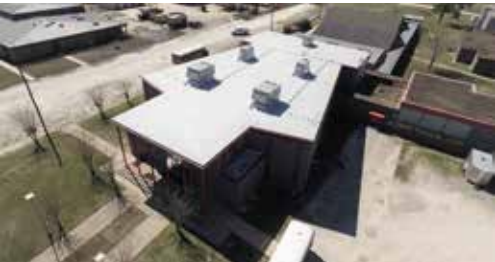
DEQUINCY HS AUDITORIUM ROOF REPLACEMENT
