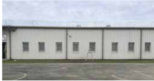
CPSD SECURITY WINDOW REPLACEMENT PH II
