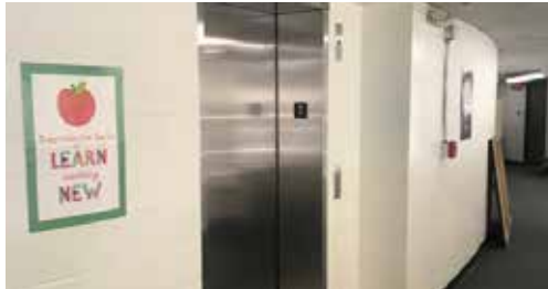
NSU NEW ELEVATOR - TEACHER'S ED CENTER
