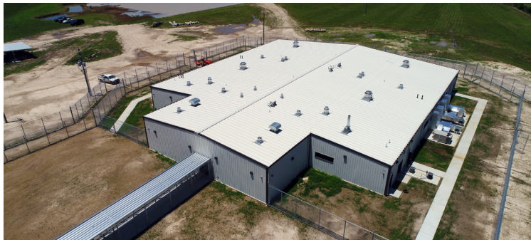
Allen Parish Detention Center
