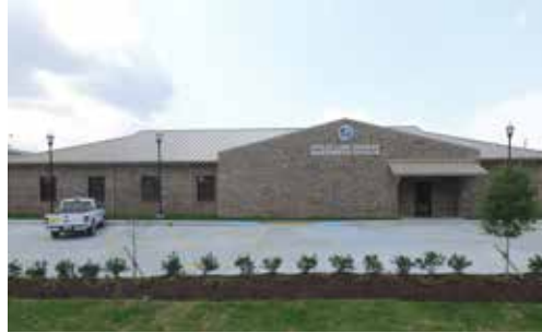
WWTP NEW ADMIN & LAB BLDG
